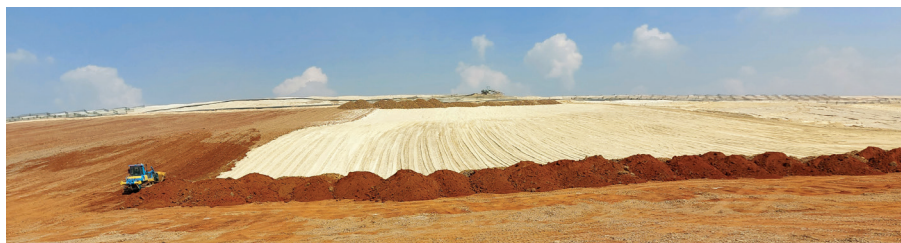
Cladding at Ergo's Brakpan/Withok TSF
