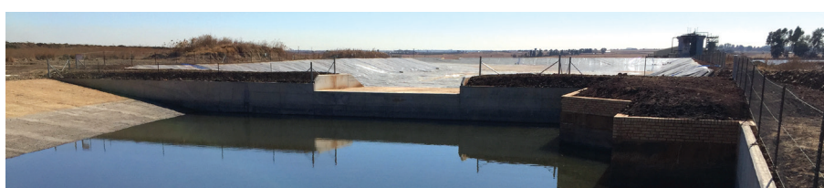
Part of silt trap at Brakpan/Withok return water dam
