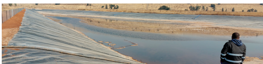
Lined return water dam at Brakpan/Withok TSF with cladded and vegetated side wall of the TSF in the background
