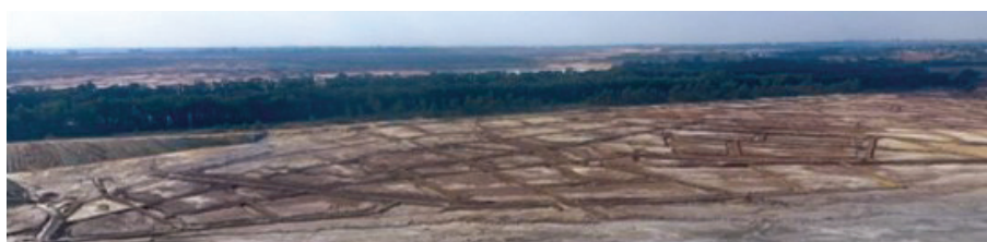
4L50 concurrent rehabilitation area: clearing to natural ground level and onsite water containment paddocks
