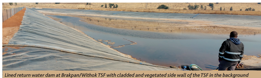
Lined return water dam at Brakpan/Withok TSF with cladded and vegetated side wall of the TSF in the background
