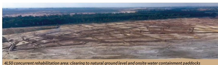
4L50 concurrent rehabilitation area: clearing to natural ground level and onsite water containment paddocks
