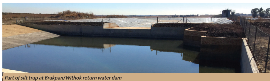
Part of silt trap at Brakpan/Withok return water dam
